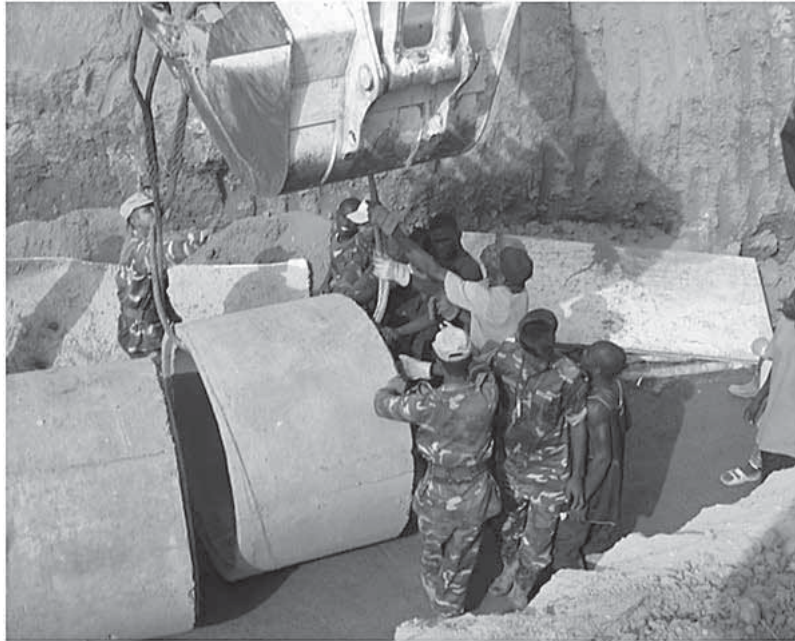
Figure 11.5. What's right with this picture? Liberian Ministry of Public Works and local personnel receive on-the-job training in culvert restoration from Bangladeshi engineers. Photo courtesy of the author.
