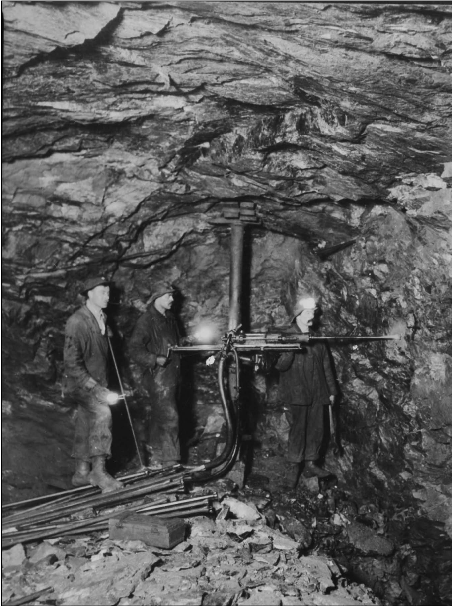
INCO Creighton Mine, method of drilling in stopes.
