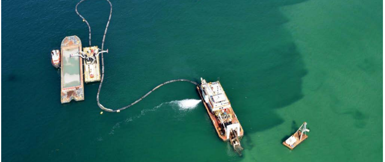
Dredger from Weeks Marine dredging a channel off Treasure Island, Florida (Photo: Dredging Contractors of America)
